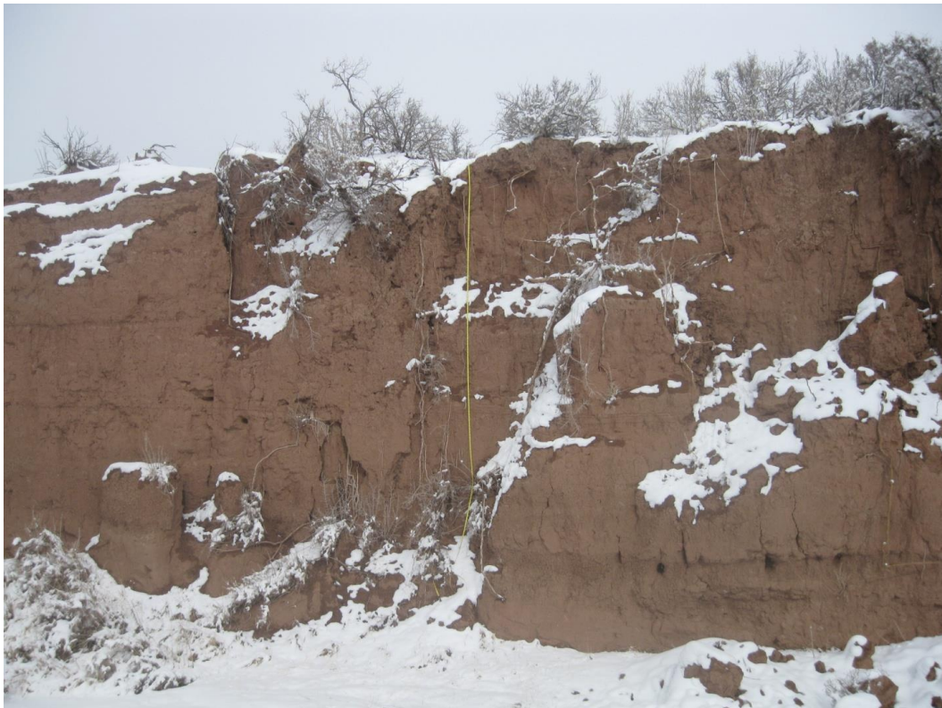
Figure 3. Photo of roots exposed in 20 foot arroyo wall.
