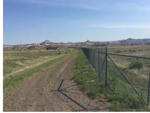
SW Corner Perimeter looking North
