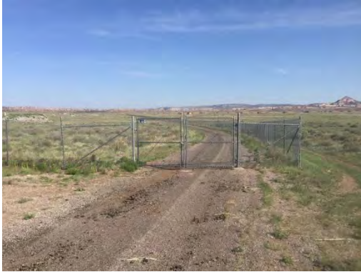
East Entrance Gate looking North
