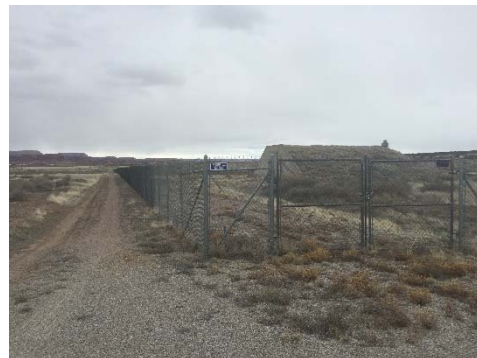
Northwest corner looking East
