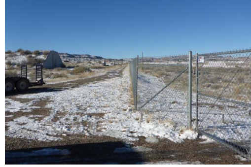
SW Corner Perimeter looking North
