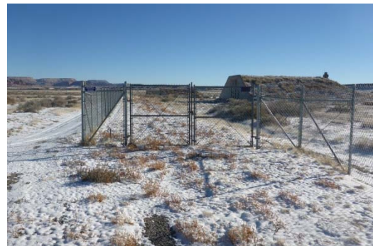
Northwest corner looking East
