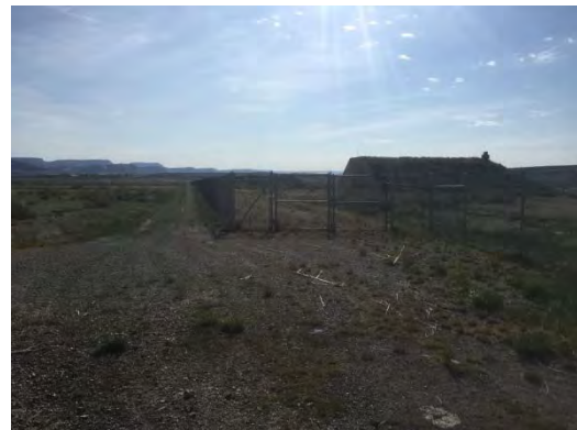
Northwest corner looking East
