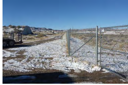
SW Corner Perimeter looking North
