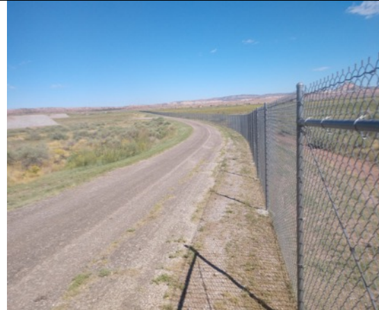
Inside perimeter of the fence looking north.
