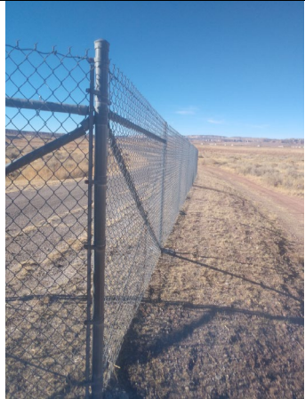
Outside perimeter of the fence looking north.
