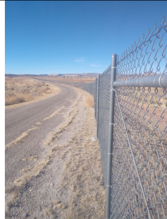
Inside perimeter of the fence looking north.
