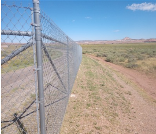
Outside perimeter of the fence looking north.
