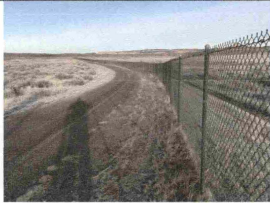
Inside perimeter of the fence looking north.
