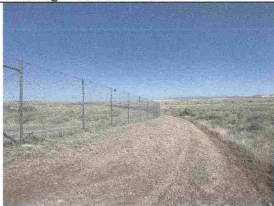
Outside perimeter of the fence looking north.
