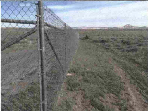
Outside perimeter of the fence looking north.
