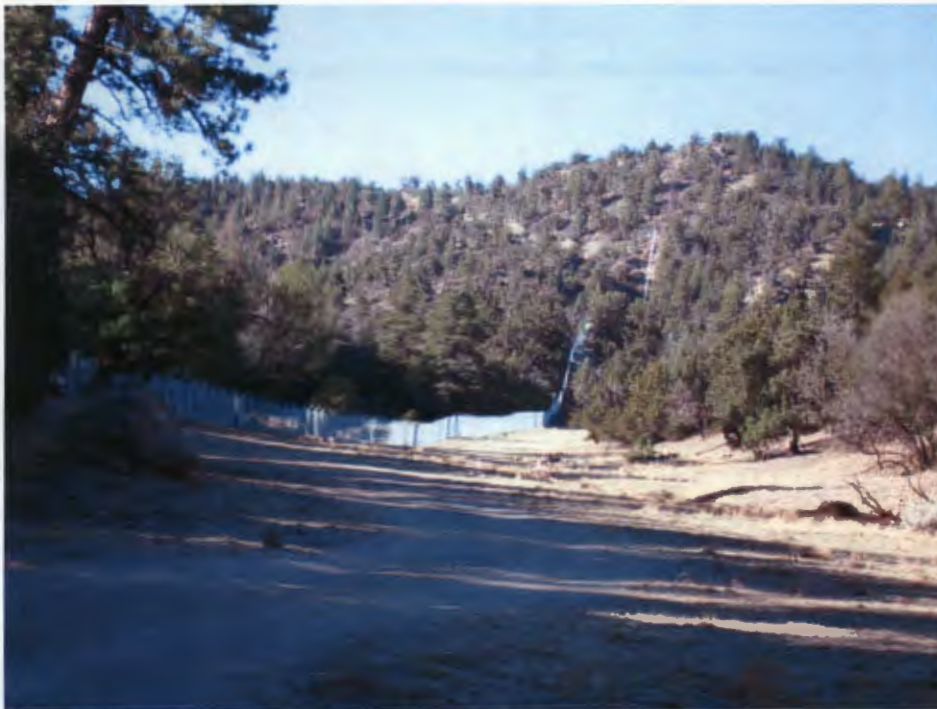
Photo 2: Chain link fence along western boundary of Parcel 3, looking south.
