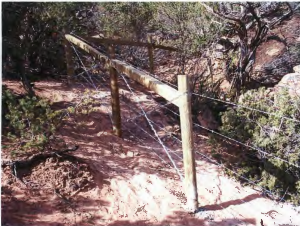
Photo 6: Barbed wire fence along northern boundary of Parcel 3, showing typical timber pull/end posts.
