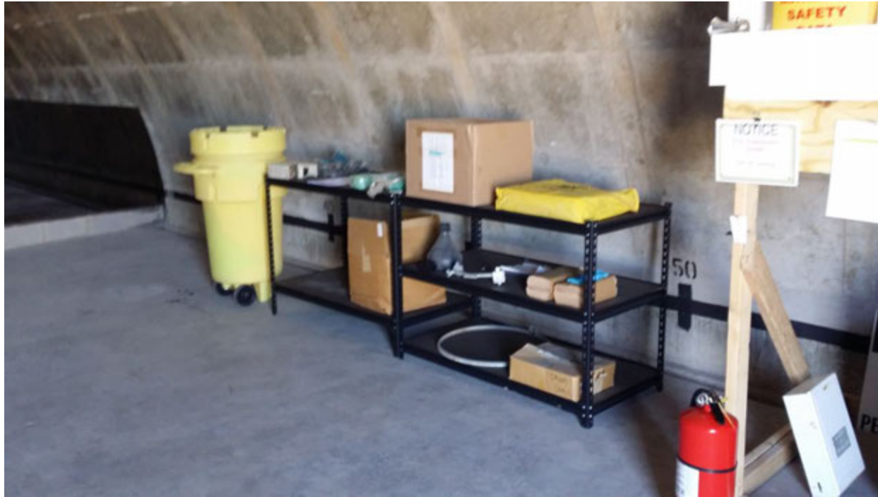
Photograph 9: Interior of Igloo B-1007, showing emergency spill supplies. Date of Photograph: 13 February 2015
