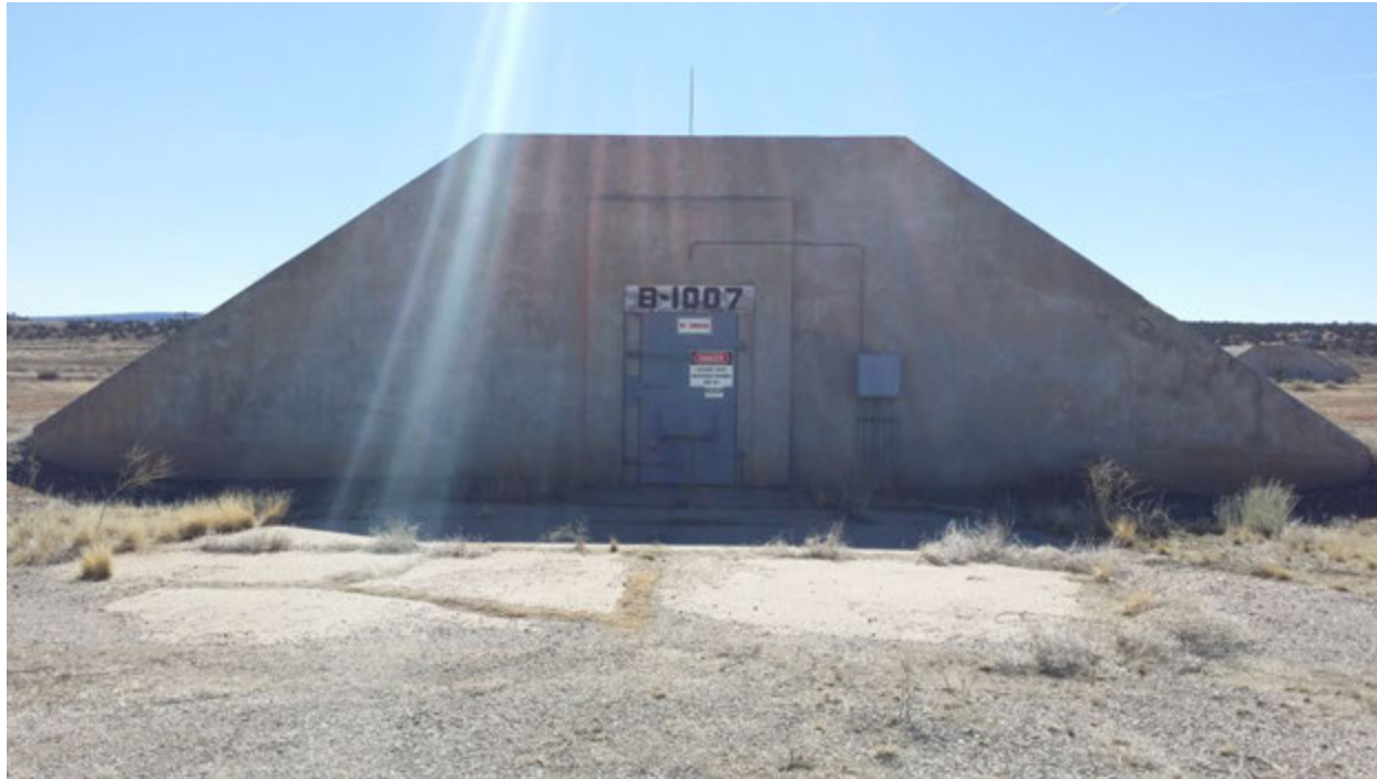
Photograph 1: Igloo B-1007 (Less-Than-90-Day holding facility) facing southeast. Date of Photograph: 13 February 2015
