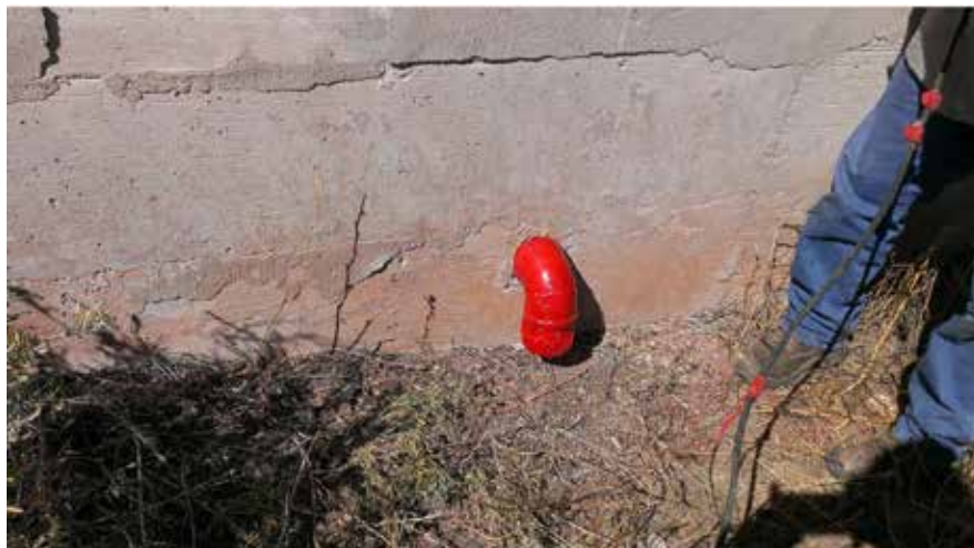
Photograph No. 2 A view of a drain pipe at Igloo C-1105.
