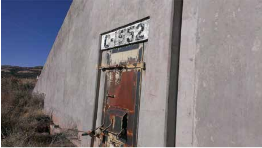
Photograph No. 13 A view of Igloo C-1552.
