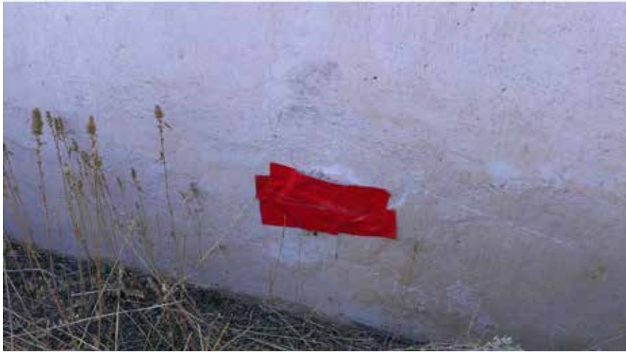
Photograph No. 7 A view of the removed drain pipe at Igloo C-1116.
