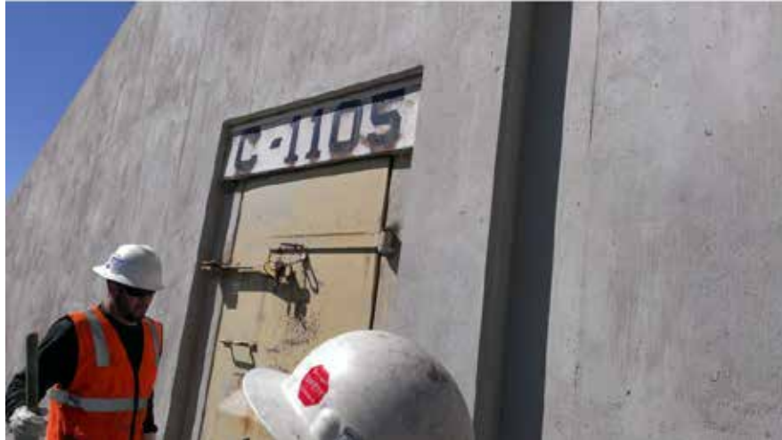
Photograph No. 1 A view of Igloo C-1105.
