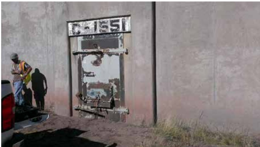
Photograph No. 8 A view of Igloo C-1551.
