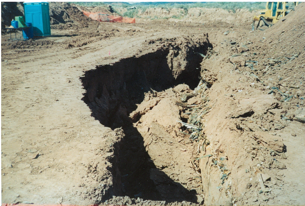
Photograph 5-4. Trench looking north at Areas K, J, I, H, and G.
