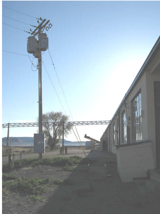
Photo 7-5: Part of AOC 75, looking east at transformers northwest of Building 528.
