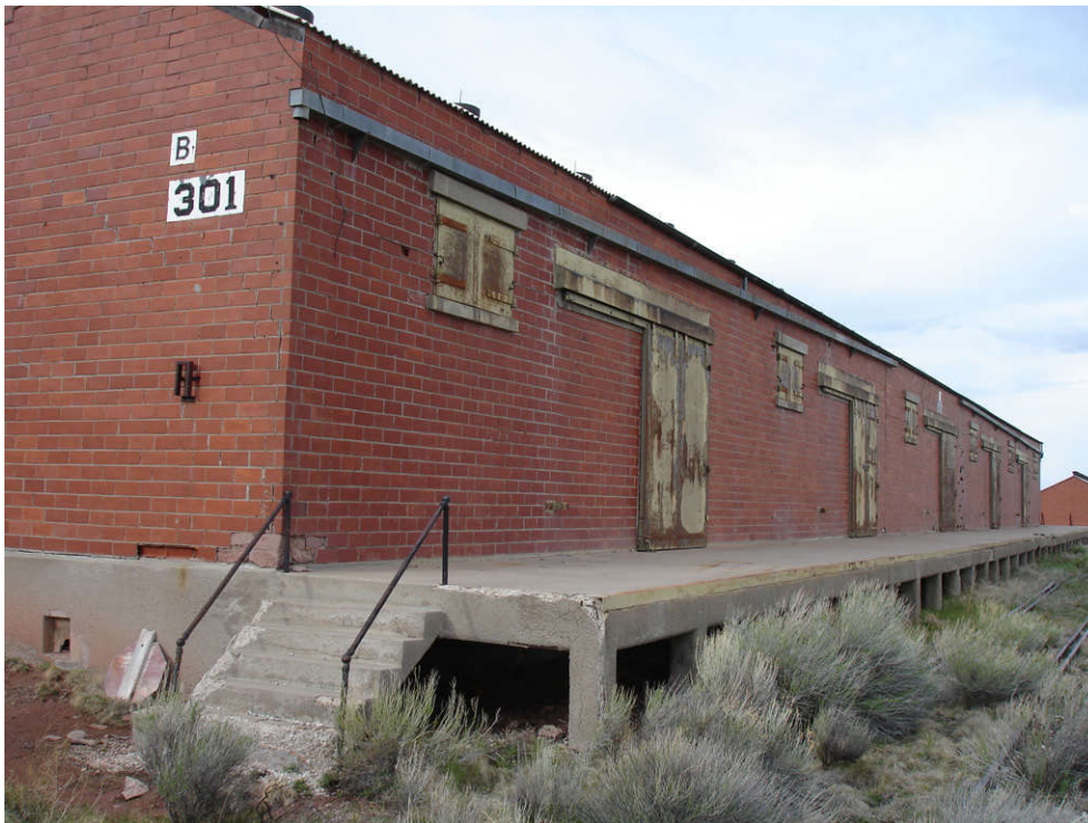
Photo 5-2: AOC 69, Building 301, Standard Magazine, looking northeast at exterior condition of building.
