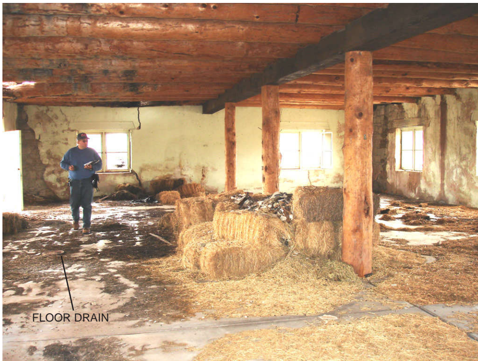
Photo 5-11: AOC 69, Building 316, looking west at interior of building.
