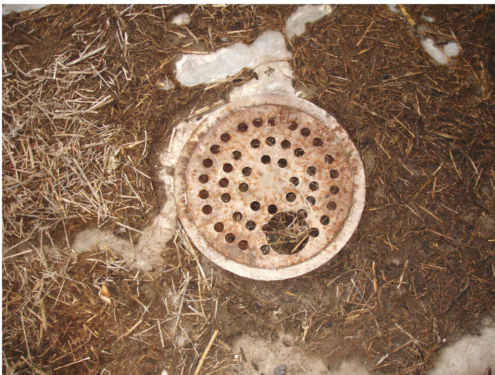
Photo 5-12: AOC 69, Building 316, showing floor drain.
