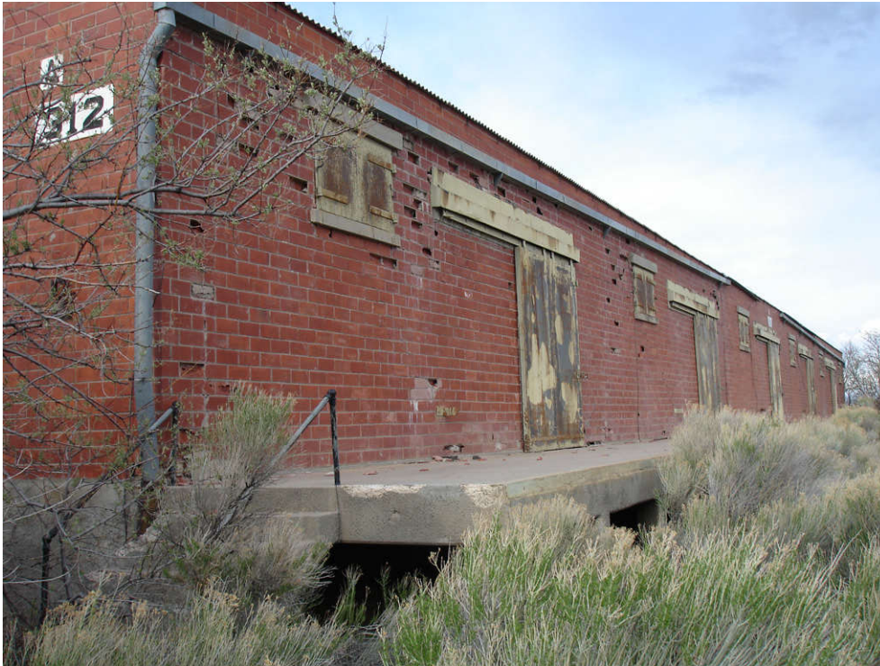
Photo 5-3: AOC 69, Building 312, Standard Magazine, looking northeast at exterior condition of building.
