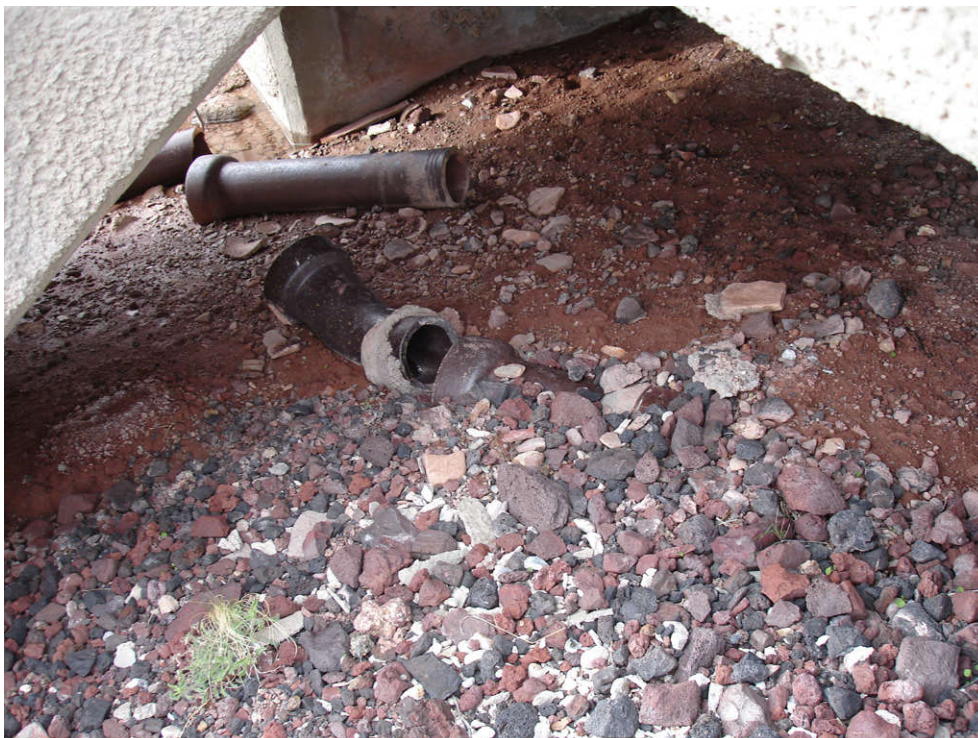
Photo 5-8: AOC 69, showing clay tile pipe rain gutter drains.
