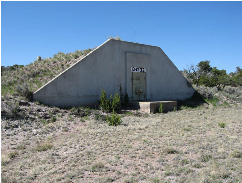
Photo 4-5: AOC 30, Igloo Block D, looking southwest at typical igloo with elevated dock.
