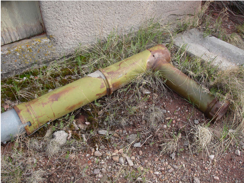
Photo 5-5: AOC 69, showing munitions shipping containers used as rain gutter drains.
