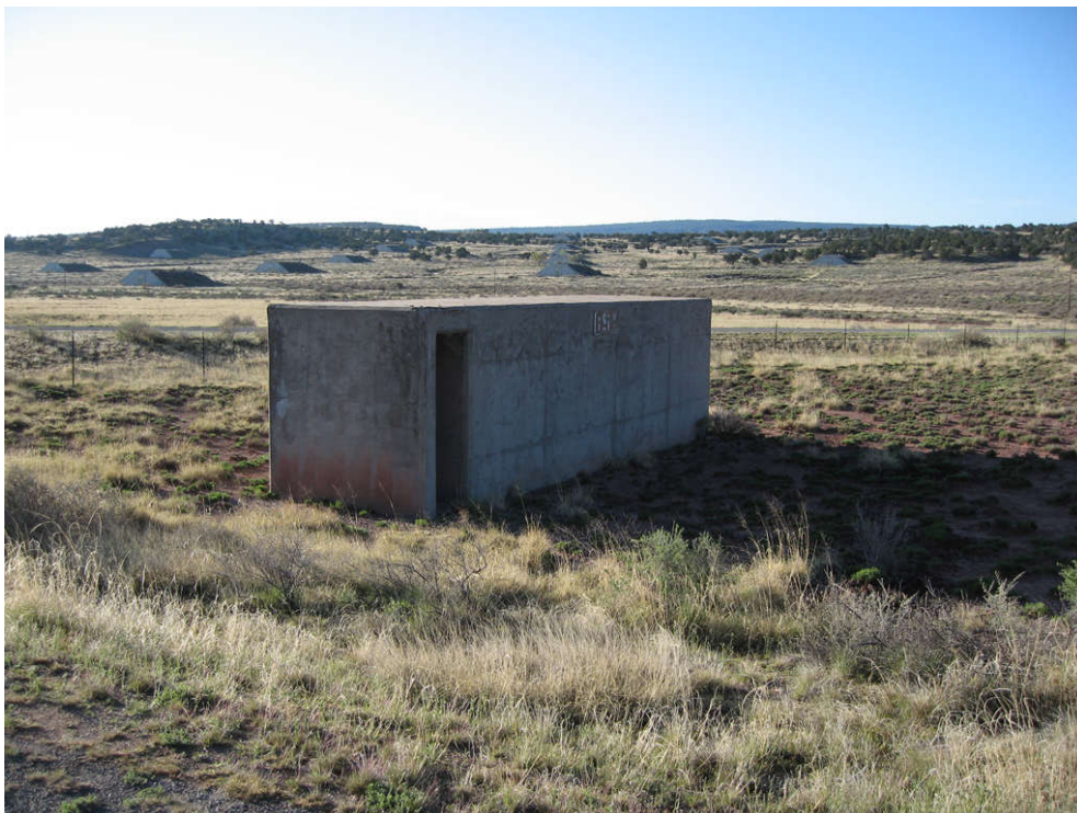
Photo 4-12: Building 317, which is a typ. concrete safety shelter.
