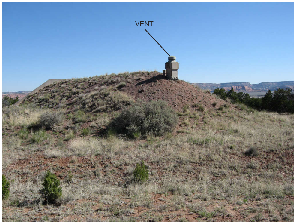
Photo 4-4: AOC 30, Igloo Block D, looking northeast at typical igloo.
