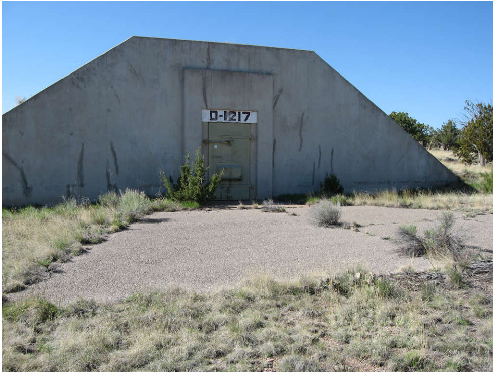
Photo 4-1: AOC 30, Igloo Block D, looking south at typical igloo.
