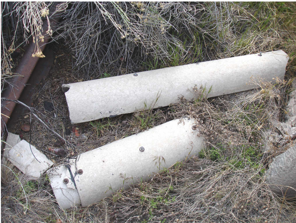
Photo 5-6: AOC 69, showing potential ACM roof tile.
