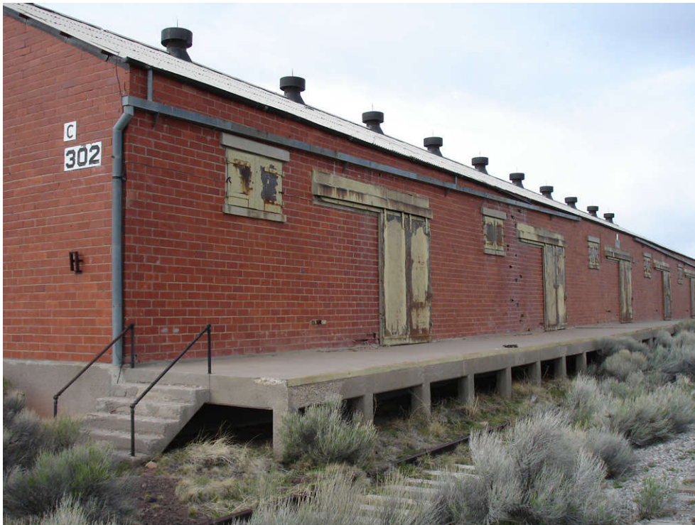
Photo 5-1: AOC 69, Building 302, Standard Magazine, looking northeast at exterior condition of building.
