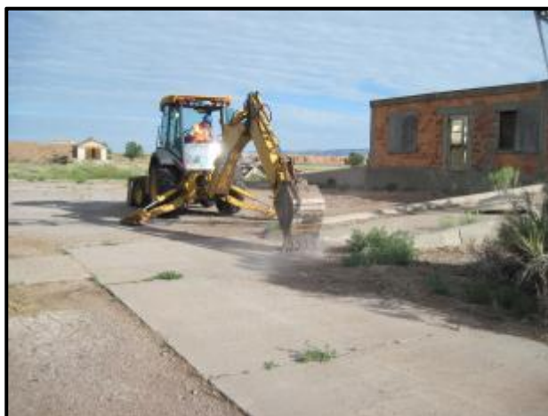
Removing concrete for sampling building 522
