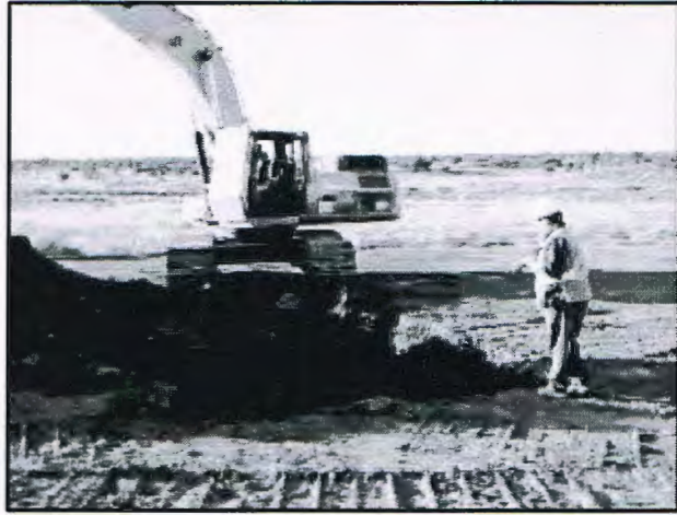
Pit sampling at building 530
