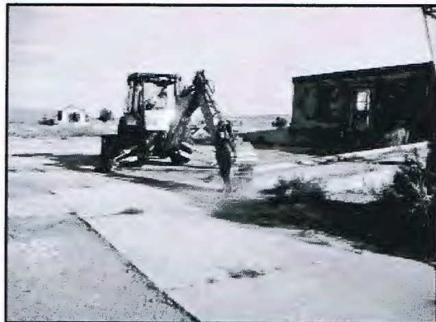
Removing concrete for sampling building 522
