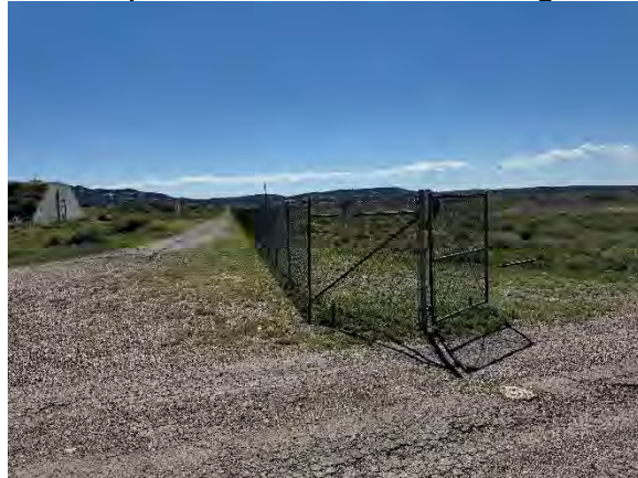
Outside perimeter of the fence looking west.
