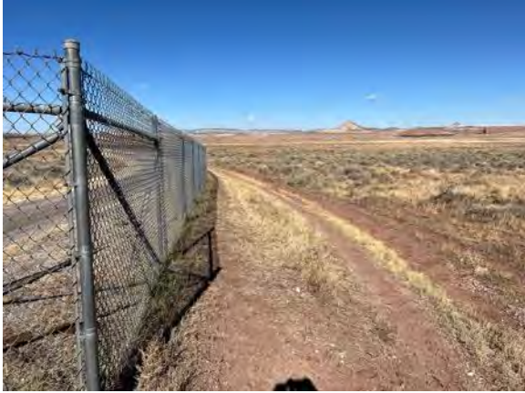
Outside perimeter of the fence looking north.
