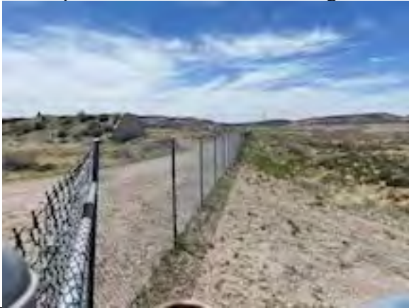
Inside perimeter of the fence looking west.
