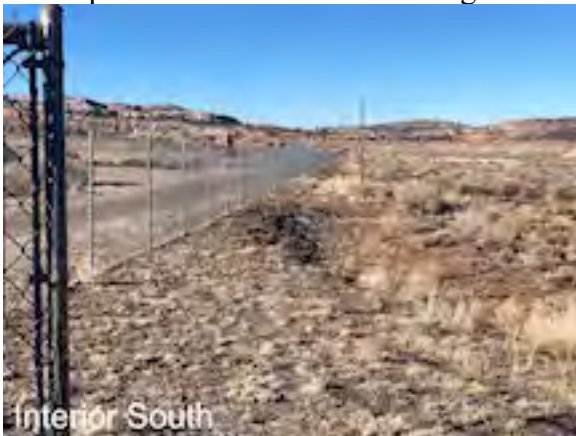
Inside perimeter of the fence looking west.
