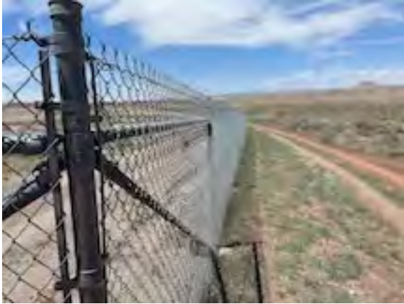
Outside perimeter of the fence looking north.
