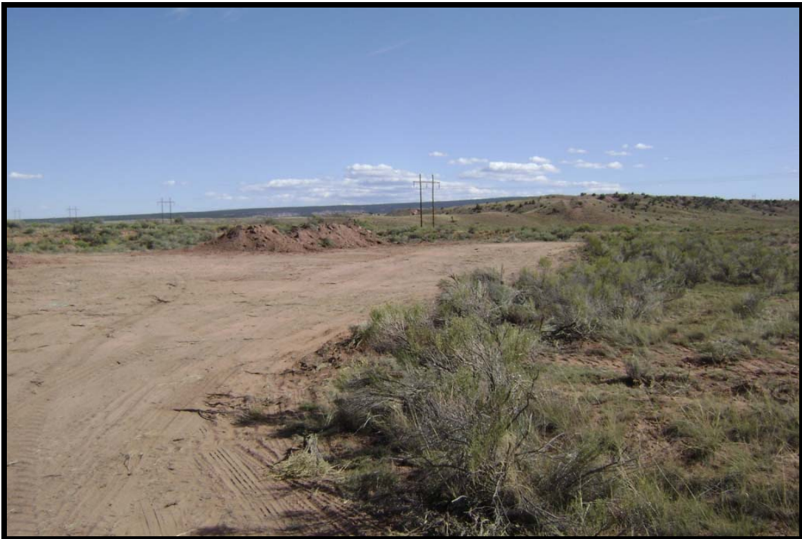
Parcel 12 / AOC 93 – Bivouac and Tank Training Area – North debris pile area removal
