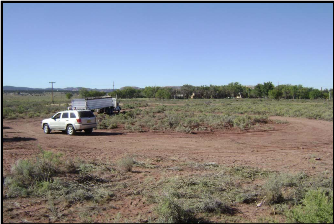
Parcel 12 / AOC 93 – Bivouac and Tank Training Area – South debris pile area removal
