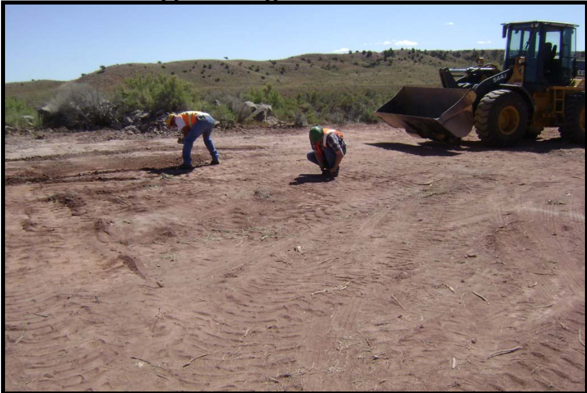
Parcel 12 / AOC 93 – Bivouac and Tank Training Area – South debris pile area removal - final sweep for remaining debris
