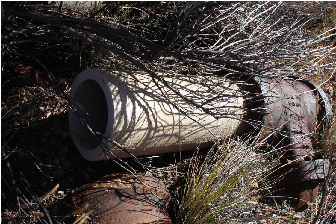
Photo 3-10: AOC 93, Bivouac and Tank Training Area, showing possible asbestos pipe.
