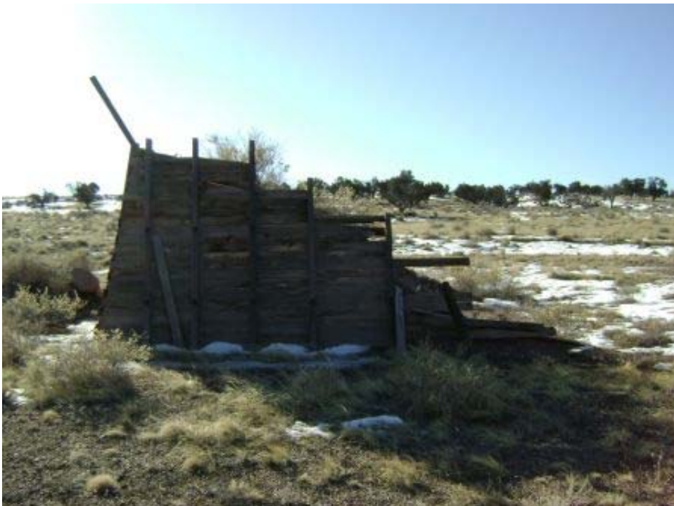
DISASSEMBLY PLANT TIMBER REVETTED BARRICADE
