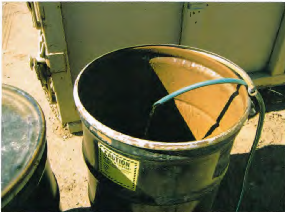
Photo 5: De-watering excavation directly into drum.
