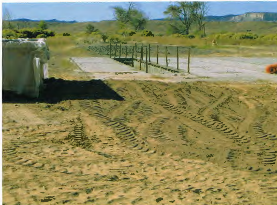
Photo 7: View to west showing backfilled excavation; completed project.
