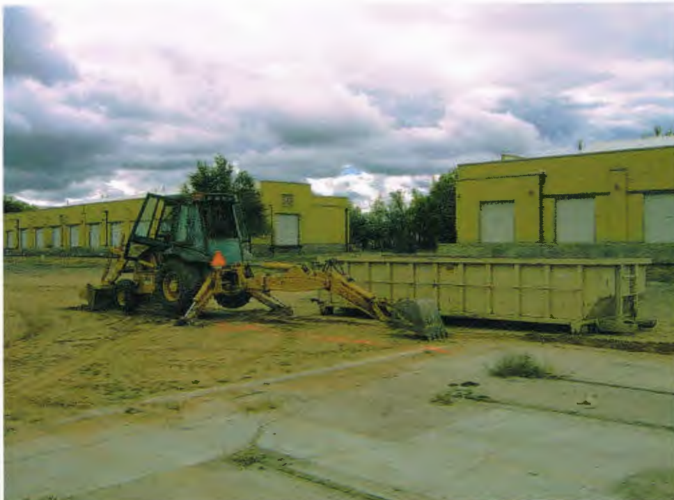
Photo 2: View to southeast showing area to be excavated.
