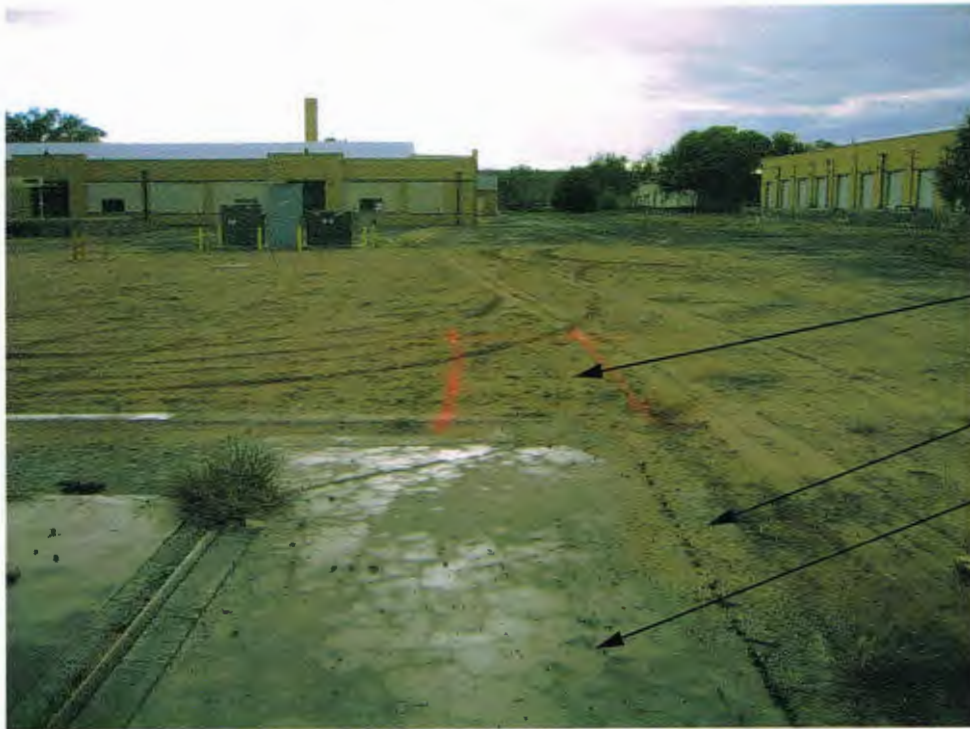
Photo 1: View to east showing existing Building 11 foundation slab, markout for excavation, and building footer.
