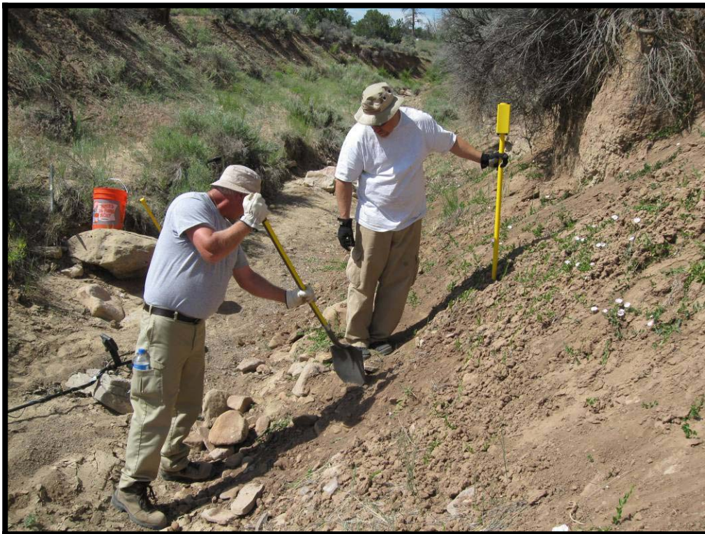
Investigating an Anomaly in Sidewall
