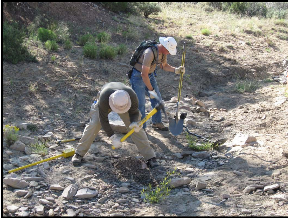
Excavating Anomaly in Arroyo Bed
