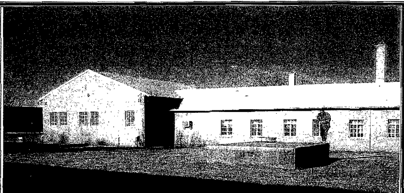
BUILDING 34 - Vault B, ID#s 17, 18, & 19
