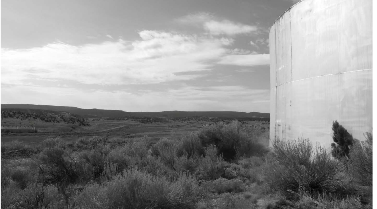
Figure 23. Storage Tank Looking Southwest.
