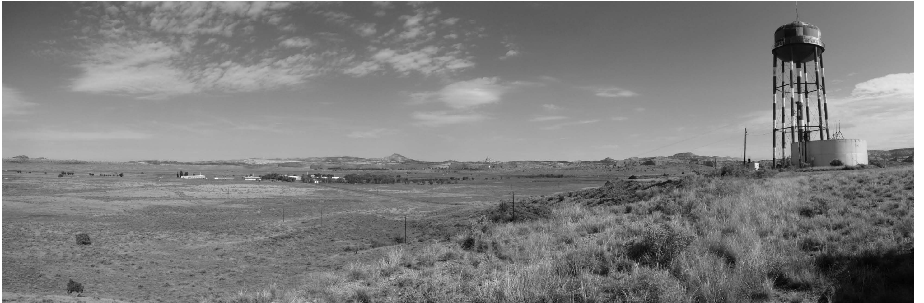
Figure26. Water Tower and Storage Tank Looking Northwest Toward Administration Area and I-40.
