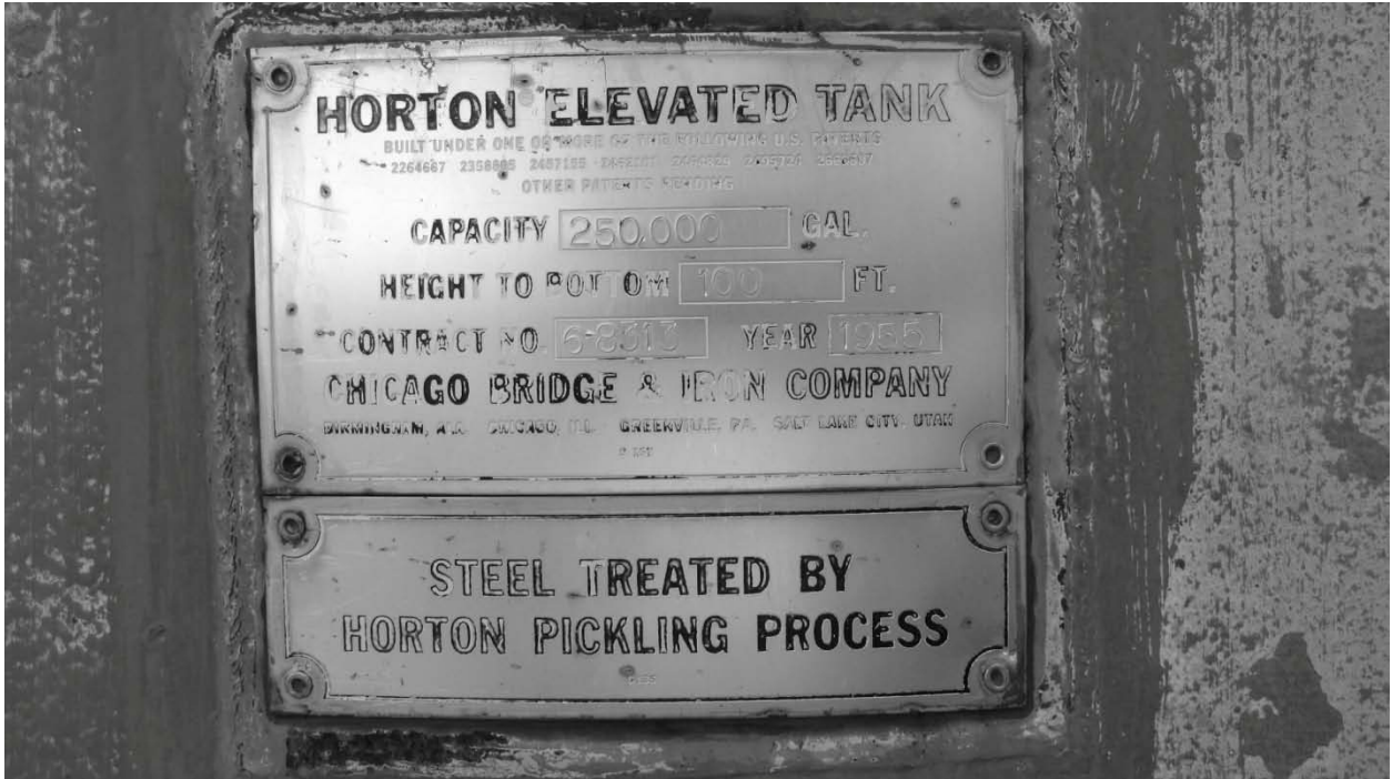
Figure 17. Water Tower. Plate Detail.
