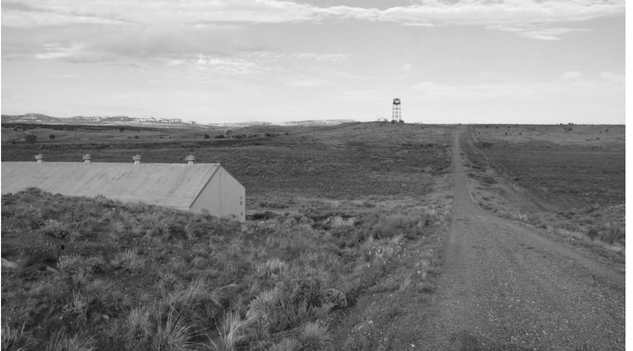
Figure 6. Water Tower Distant View from Magazine Area Looking West.
