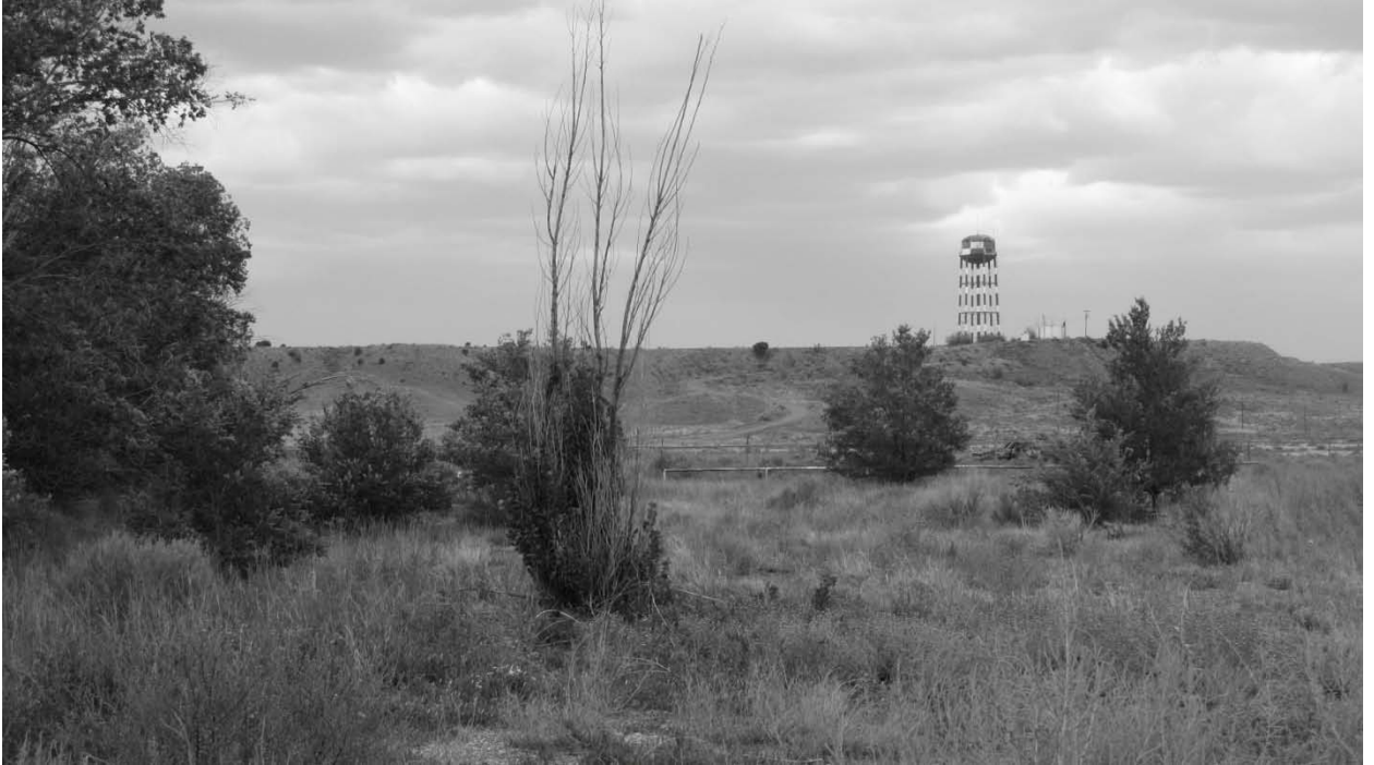
Figure 5. Water Tower Distant View from Admin Area Looking East.
