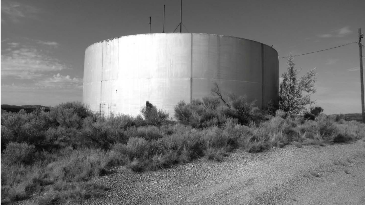
Figure 18. Storage Tank Looking West.
