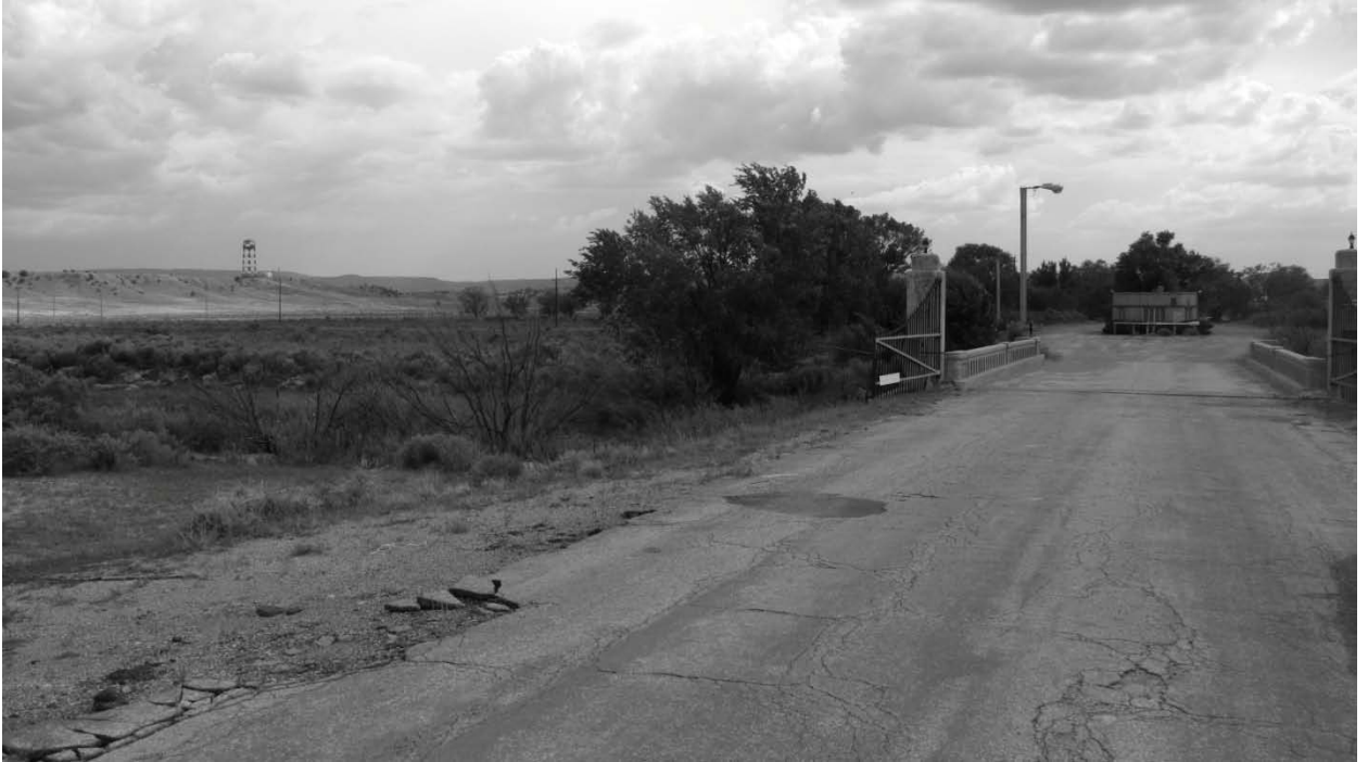
Figure 4. Water Tower Distant View From Admin Area Looking South.
