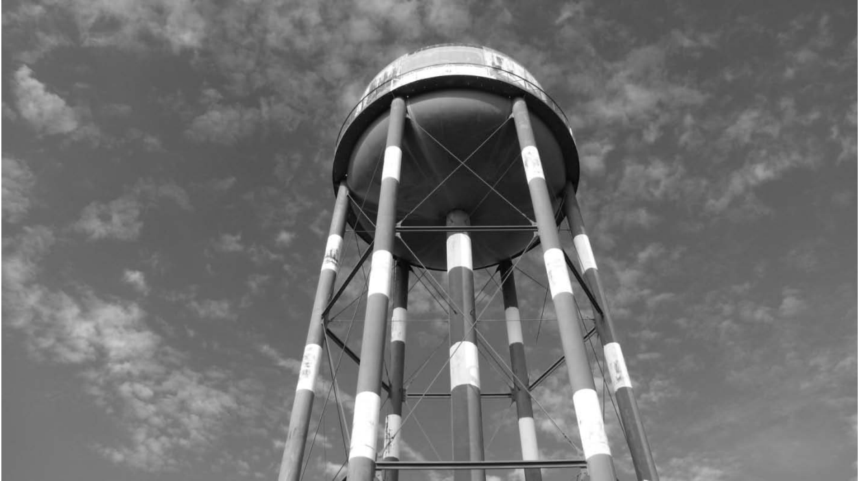
Figure 10. Water Tower. Detail.
