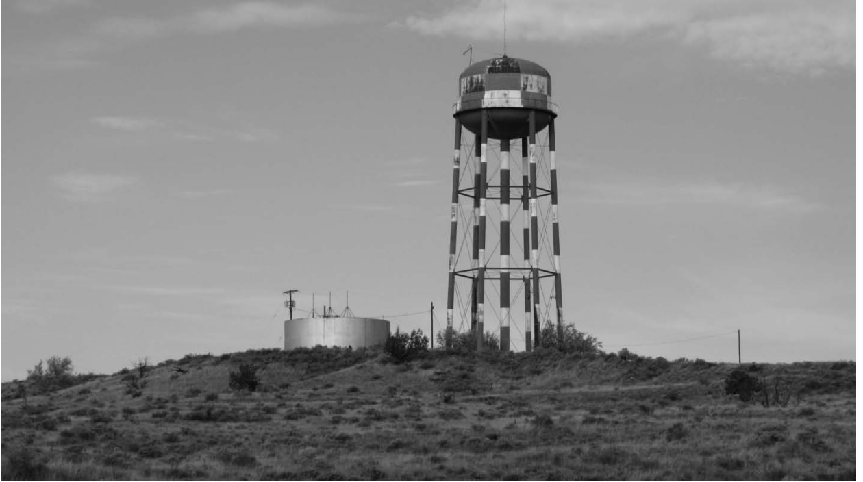
Figure 9. Water Tower and Storage Tank Looking West.
