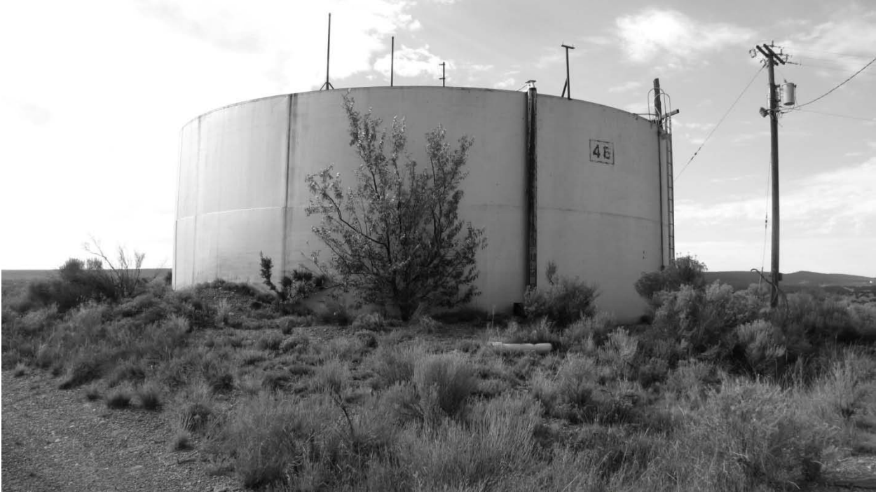
Figure 19. Storage Tank Looking South.
