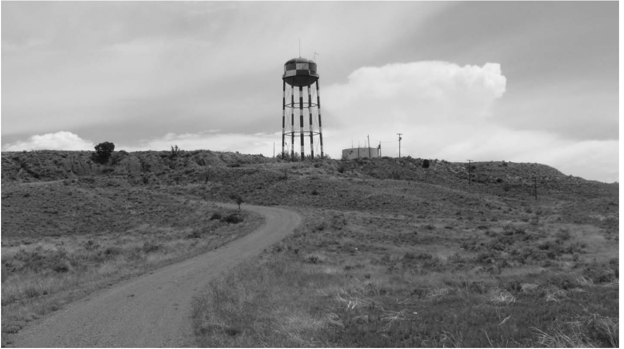
Figure 7. Water Tower and Storage Tank Looking West.
