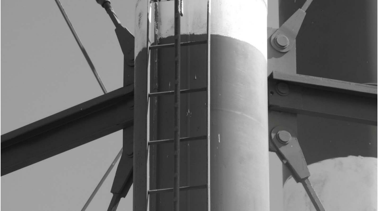
Figure 13. Water Tower. Ladder Detail.
