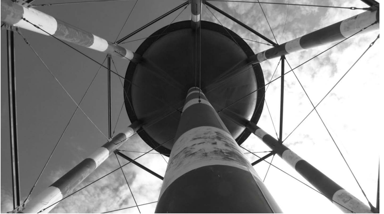
Figure 16. Water Tower. View from Bottom.
