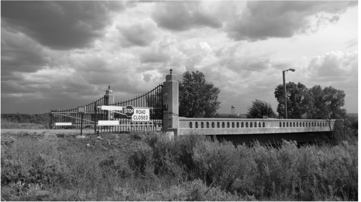
Figure 3. Water Tower Distant View from Admin Area Bridge Looking Southeast.
