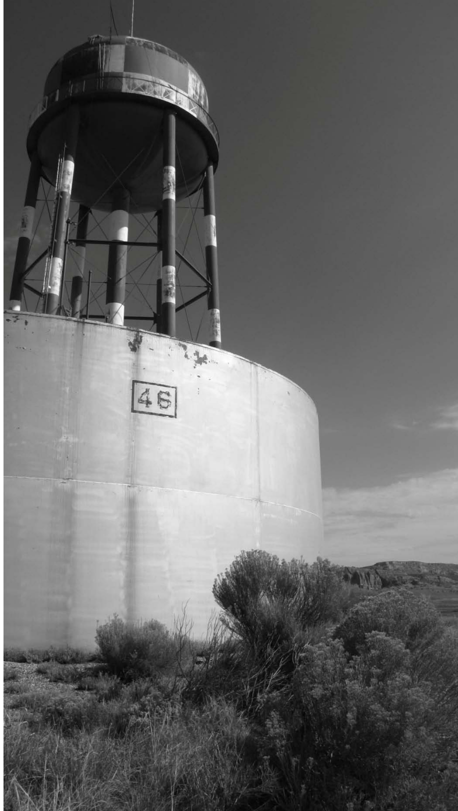
Figure 24. Water Tower and Storage Tank Looking North.
