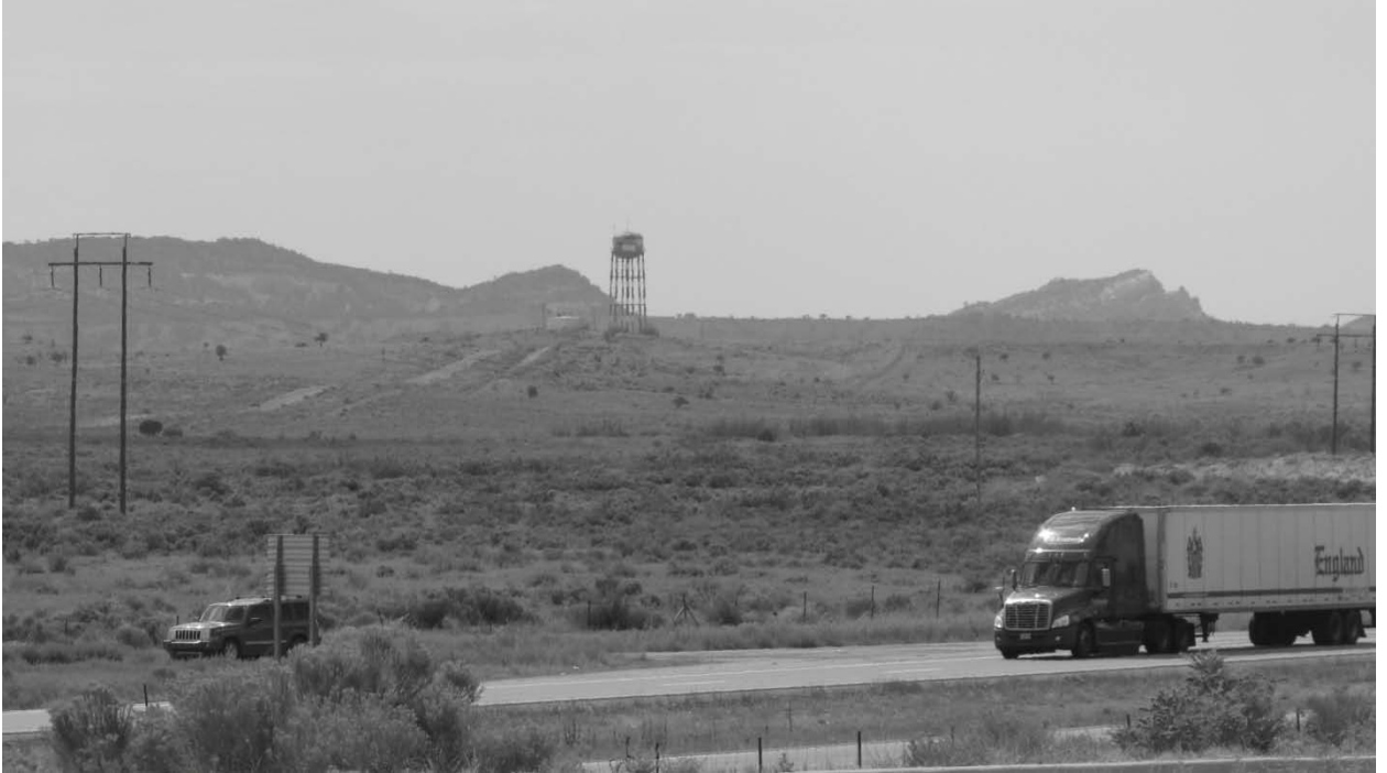
Figure 2. Water Tower Distant View from I-40 Looking Southwest.
