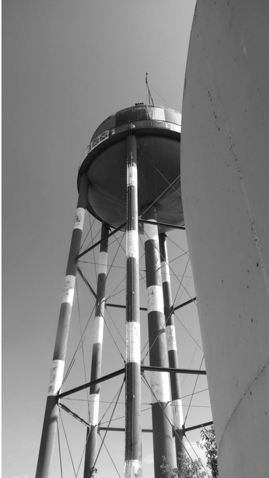
Figure 25. Water Tower and Storage Tank. Detail.
