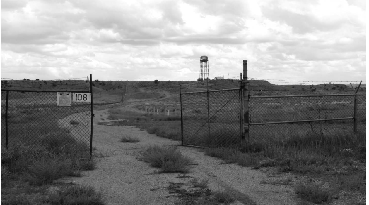
Figure 8. Water Tower and Storage Tank from Admin Area Looking West.
