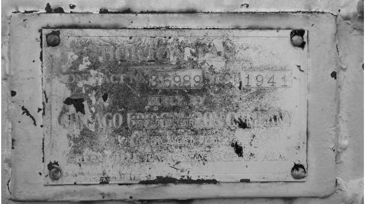
Figure 21. Storage Tank. Plate Detail.
