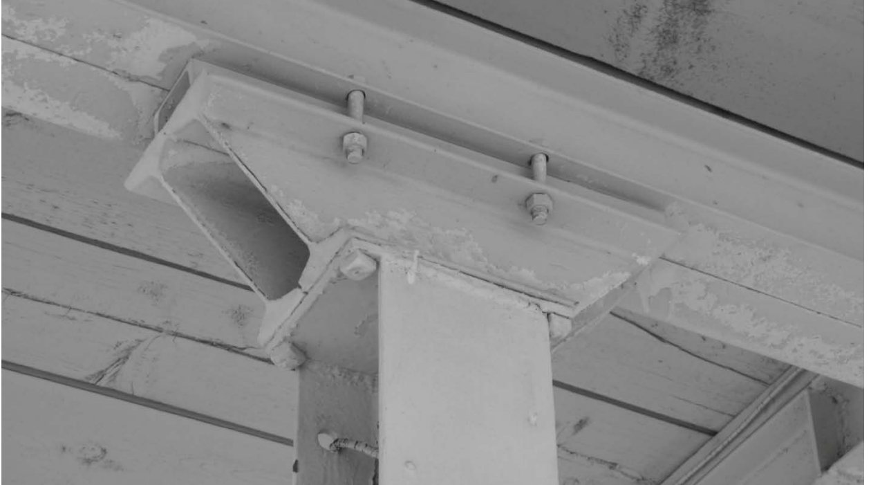
Figure 6. Gas Station Canopy Column Detail.
