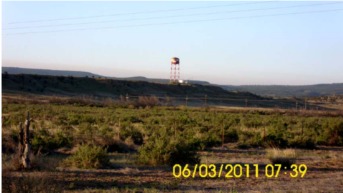
Figure 1. Structure 53. Distant View from I 40.
