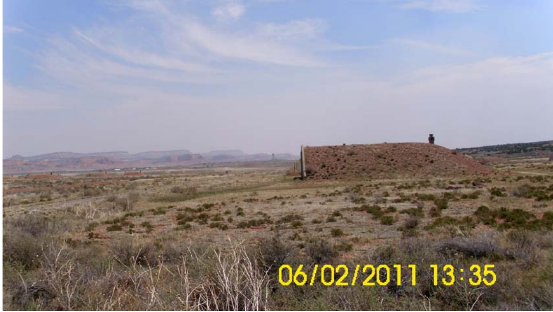
Figure 3. Structure 53. Distant View from Magazine Area.
