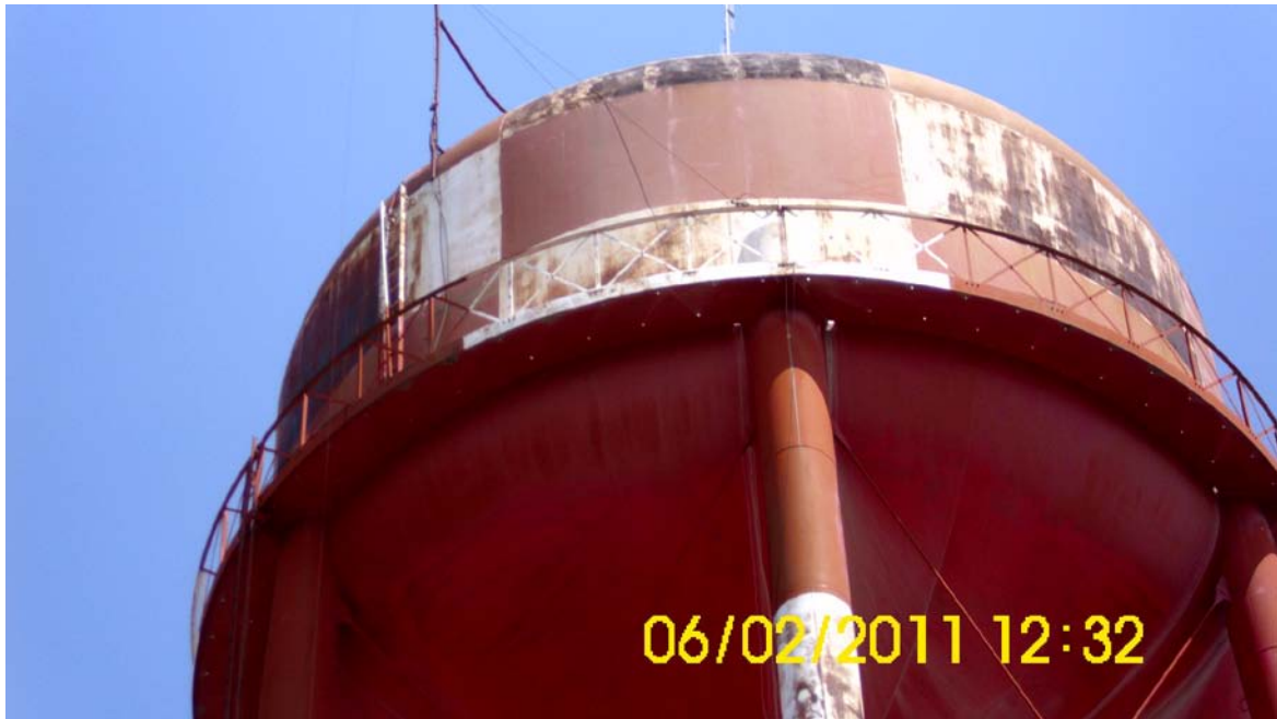
Figure 7. Structure 53. Water Tank Detail.
