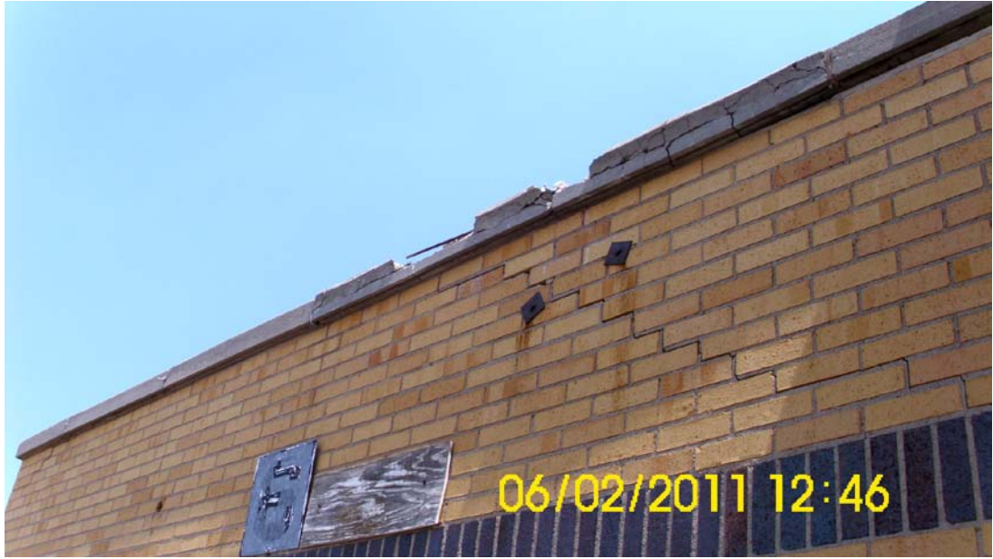
Figure 12. Structure 6. Gas Station. Detail of Structural Damage.
