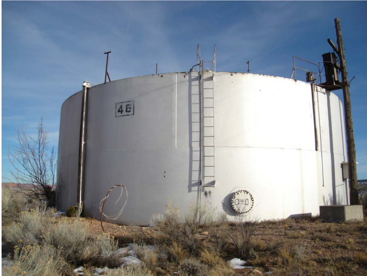
Figure 6. Structure 46. Water Tank.
