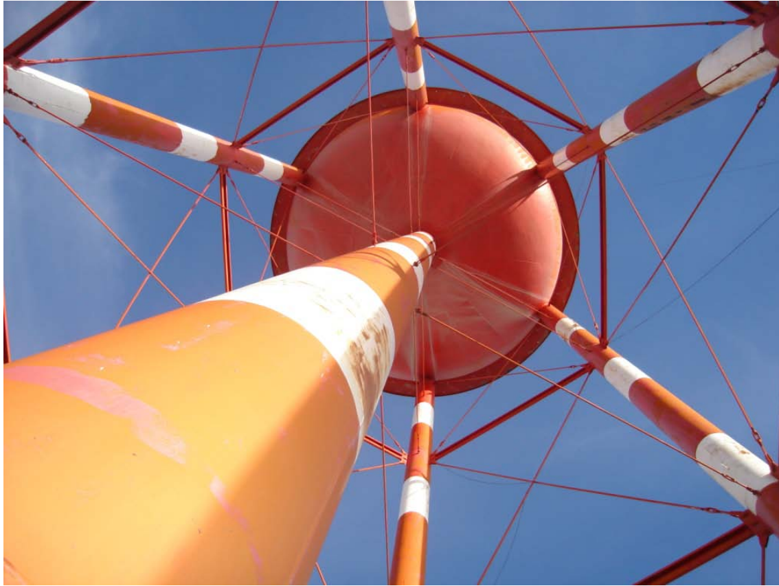
Figure 8. Structure 53. Water Tank Detail.
