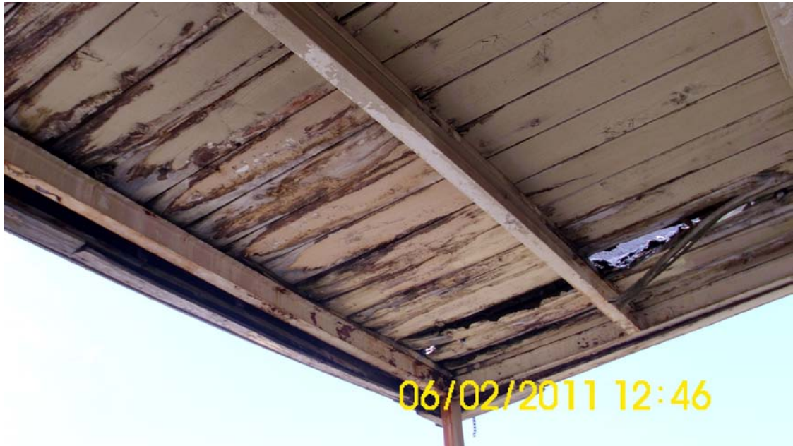
Figure 13. Structure 6. Gas Station Canopy Detail.
