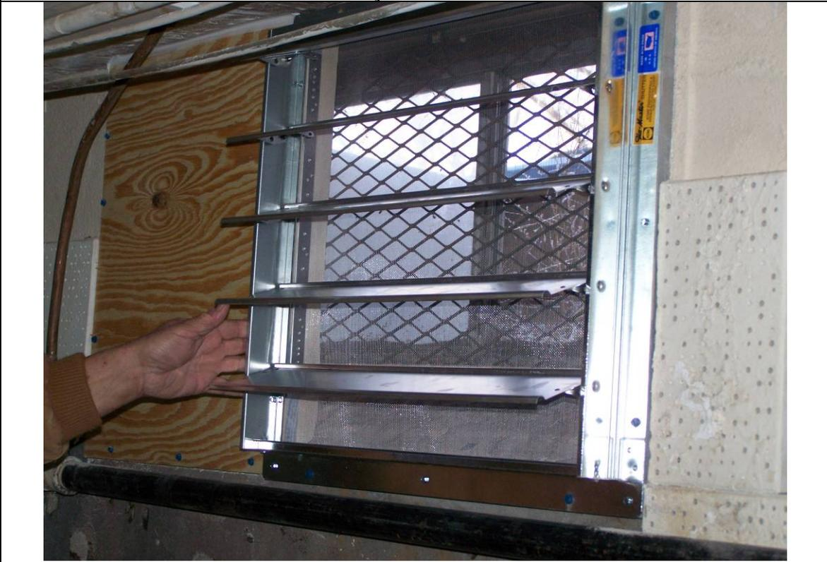
Thermostatically Controlled Air Intake Louvers
