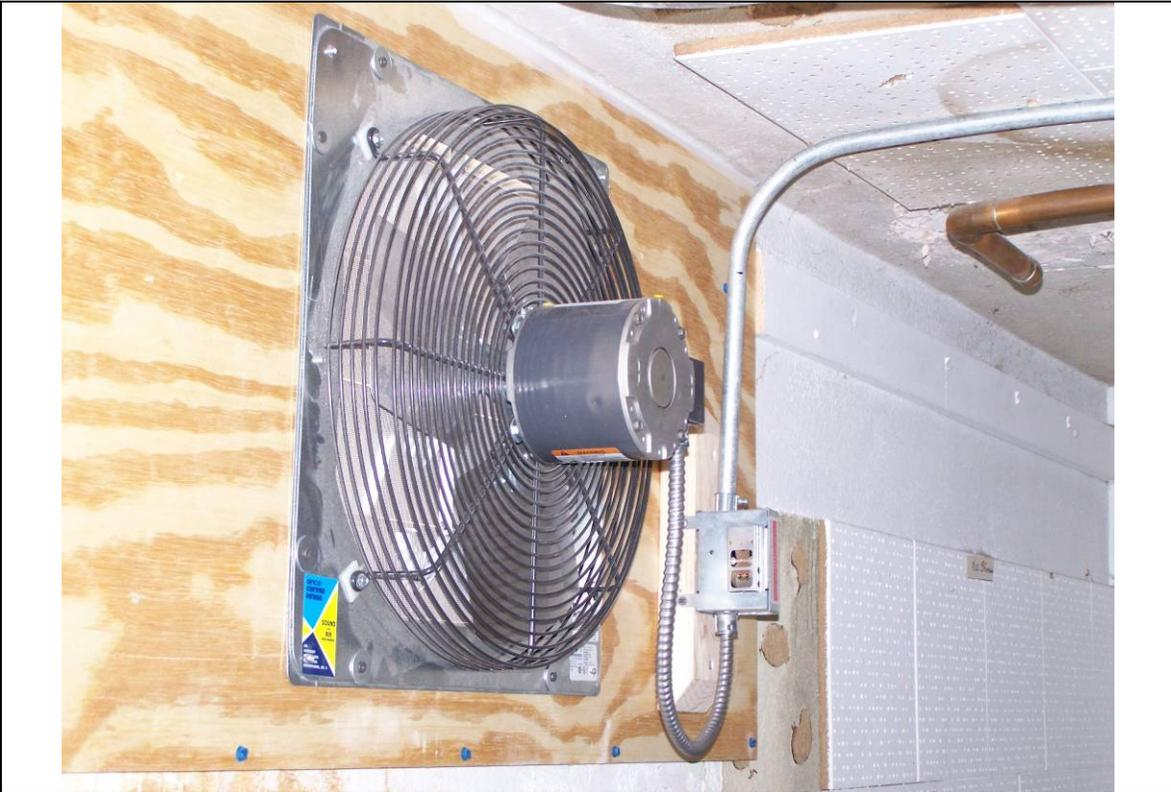
Thermostatically-Controlled Exhaust Fan
